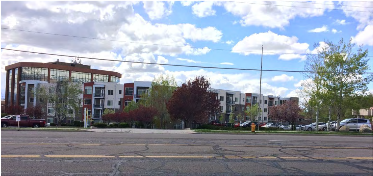
View of the north end of the subject property, which contains a parking lot for the current office building on the subject property. The adjacent credit union parking lot can be seen on the right.
