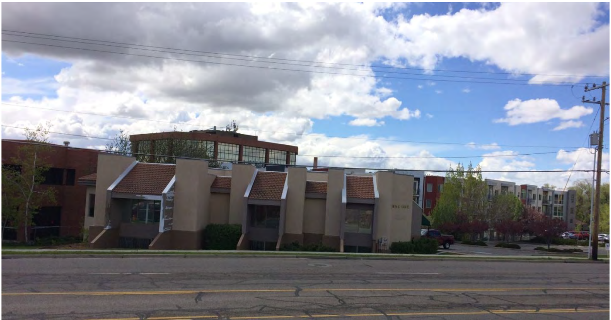
Close up view of existing two-story office building on the south end of the subject property.
