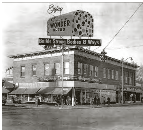
Historical photo of the Sugar House Business District at 2100 South and 1100 East
